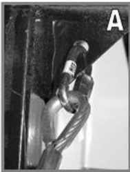
A Quick Link cable hook-up at top of the door frame
