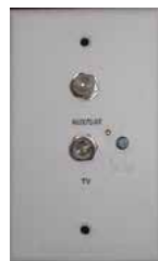
Antenna Power Supply
