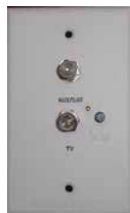
Antenna Power Supply
