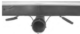
Black/Grey tank drain & valves
